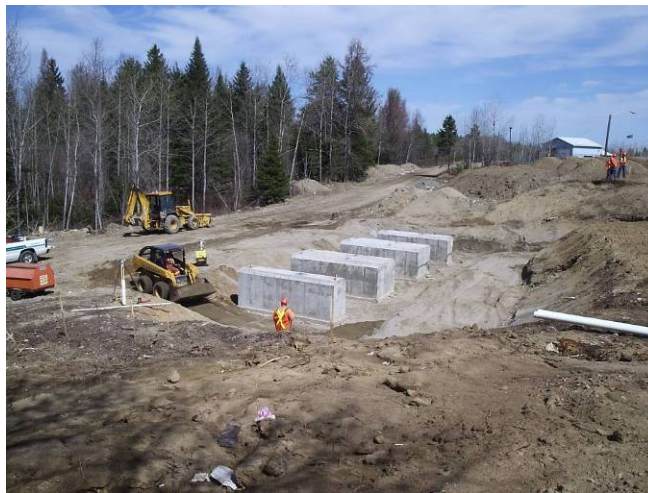
Photo 2 – Concrete Footings for Transtors
