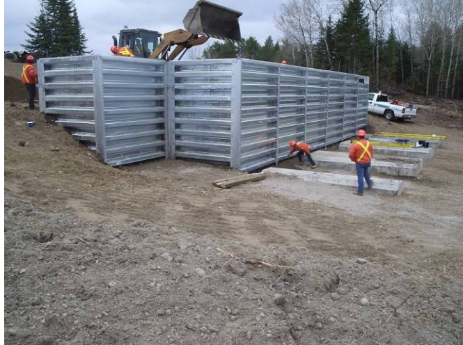
Photo 3 – Bin Wall Installation
