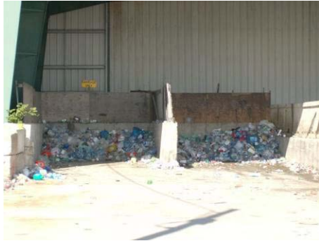
Photo 8 - Container Storage Area
