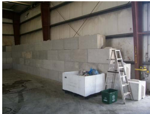
Photo 4 – Fibre Storage Area showing new retaining walls
