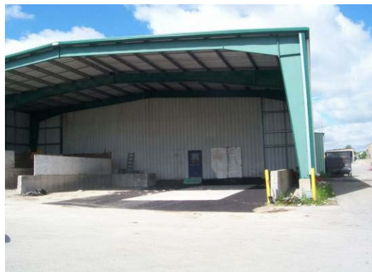
Photo 5 – Preparation of Compactor Area
